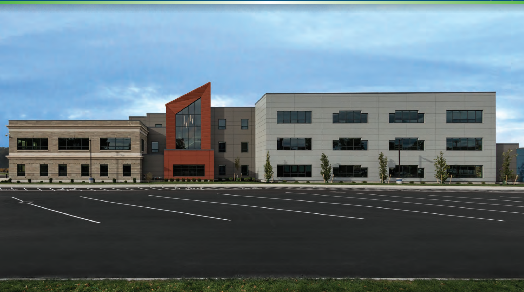
South Elevation - Offering vibrant colors and patterns the multi-colored linear insulated metal panels provide a transformation from the traditional brick and mortar schools of yesterday and offers a contemporary, energetic design. Large windows depict the program's rhythm, while the solar controlled glazing reduces solar heat gain while still allowing visible daylight transmittance and unhindered views.
