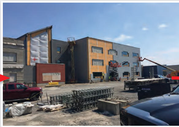
JUNE 2018 Installation of Insulated Metal Panels
