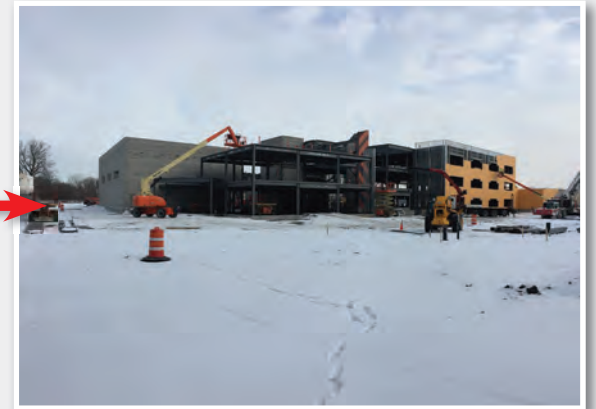
FEBRUARY 2018 Metal Studs & Exterior Sheathing
