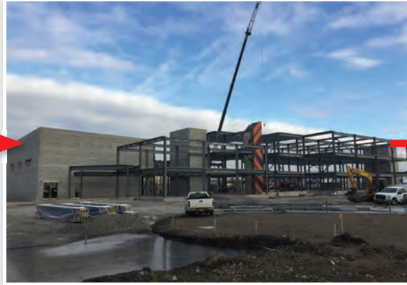
DECEMBER 2017 Steel & Masonry Erection
